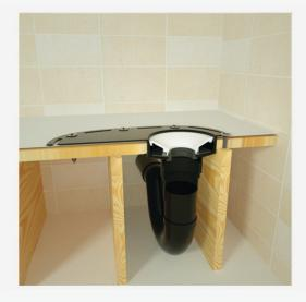
**4.** Secure the drain body to the wood floor using screws or cement.
