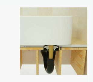
**9.** Carefully insert the bathtub tailpiece into the drain body until the bathtub is in place.
