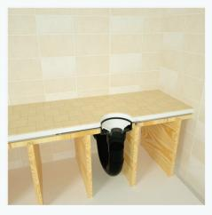
**5.** Do not obstruct the hole of the drain body. Be sure to leave enough space around the drain body.
