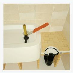
7. Install the piece to the tub's waste and overflow. Ensure the measurement between the base of the drain and P-trap will fit the tail piece.
