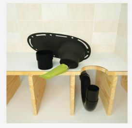
**2.** Measure and cut a ABS or PVC piece as needed to ensure a secure connection with the P-trap below. Note that the drain body has an outlet of 2" (a coupling reducer of 1  $^{1/2}$ " is included).
